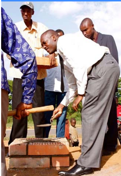
Above: Appollinaire Mplikanyi of the National Youth Council lays the first stone at the groundbreaking ceremony. Below: The MCR community center as of January 2009.
