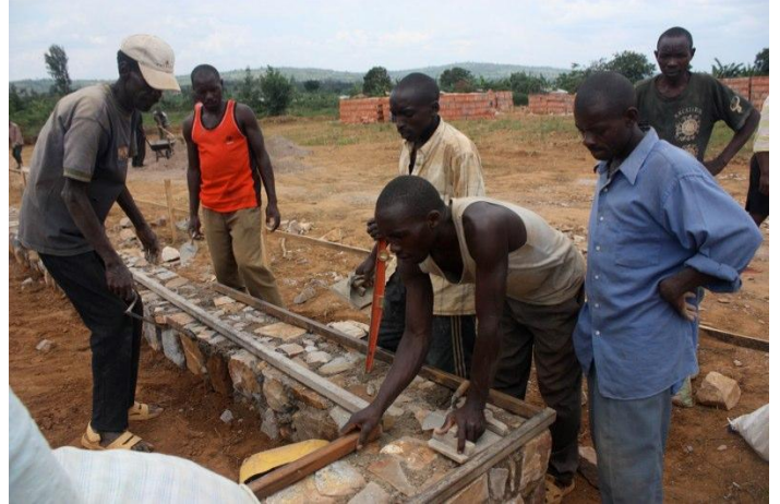
NTAMARA, RWANDA- Construction thus far on the Community Center
