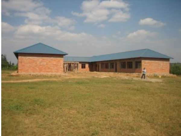
NTAMARA, RWANDA- Rwandans work on the construction of the community center
